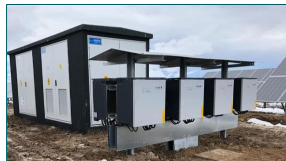
Fig.2: virtual central inverter solution
